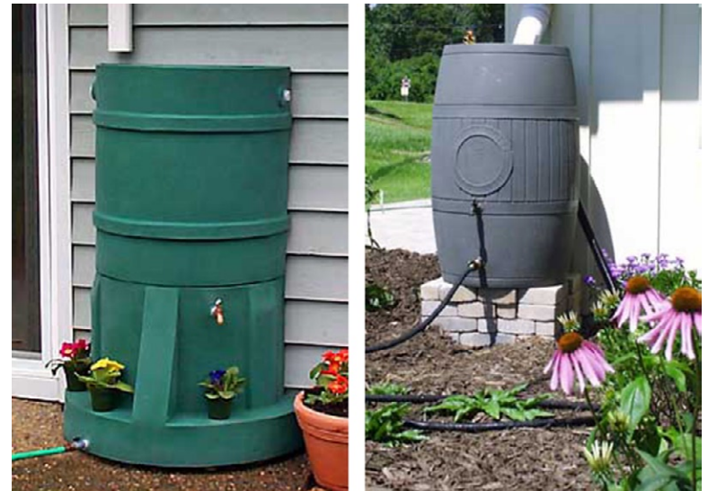
Rain barrels collect roof water for irrigation and reduce runoff ( www.rainsaverusa.com , www.clearwaterconservancy.org )
