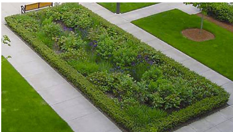
Infiltration basin in a courtyard (City of Portland 2004 Stormwater Management Manual)
