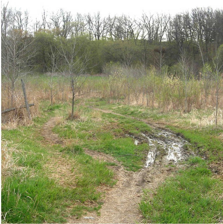
Depressions in level surfaces hold water, causing trail widening
