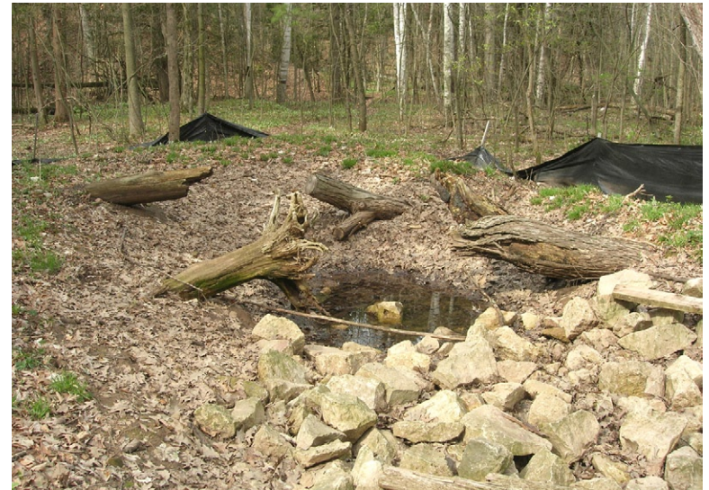
Lower discharge basin from a wet detention pond at the Royal Woods Subdivision off Huron Road
