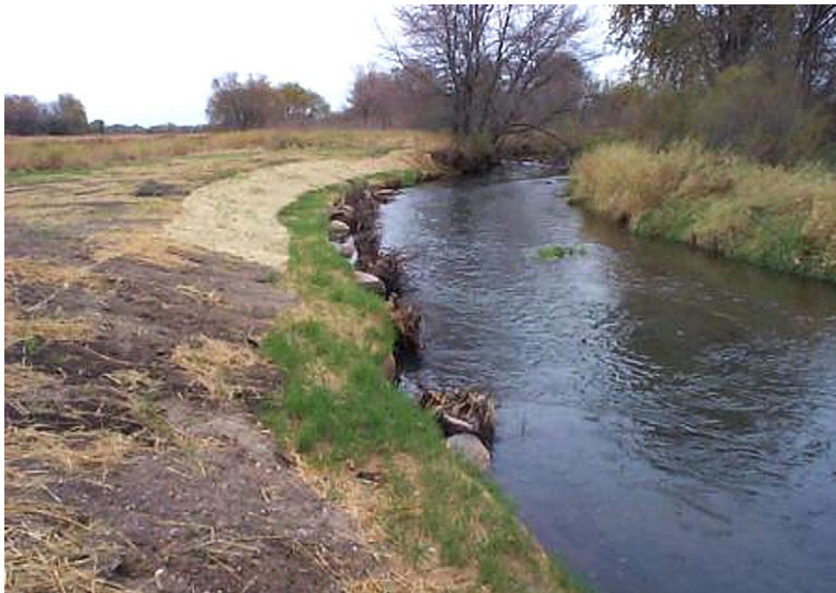
Root wads, boulder vanes, and erosion matting on the Vermillion River (Friends of Mississippi River, www.fmr.org )
