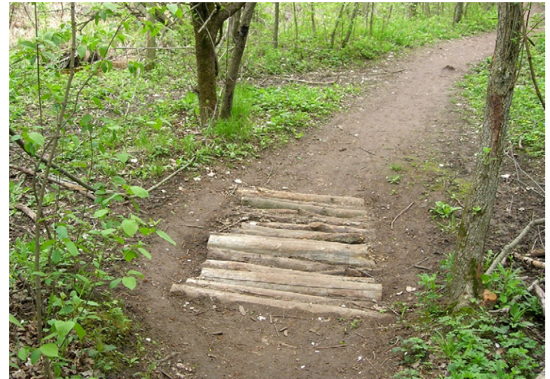
Example of preferential cutting around a corduroy trail repair
