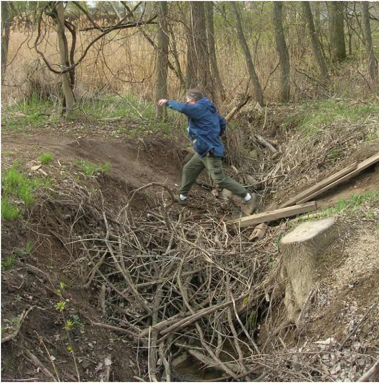
Potential tributary erosion demonstration site near Danz Avenue
